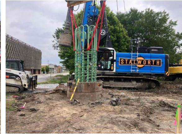
***North Segment Activities: Substructure work for elevated structures including installation of bents, caissons, piers, and foundations***
