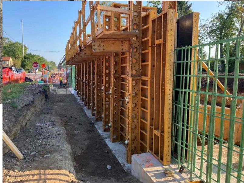
***South Segment Activities: Retaining wall construction, removal and storage of existing ped bridge at the Little Cal River, preparations for Bridge 107 construction***
